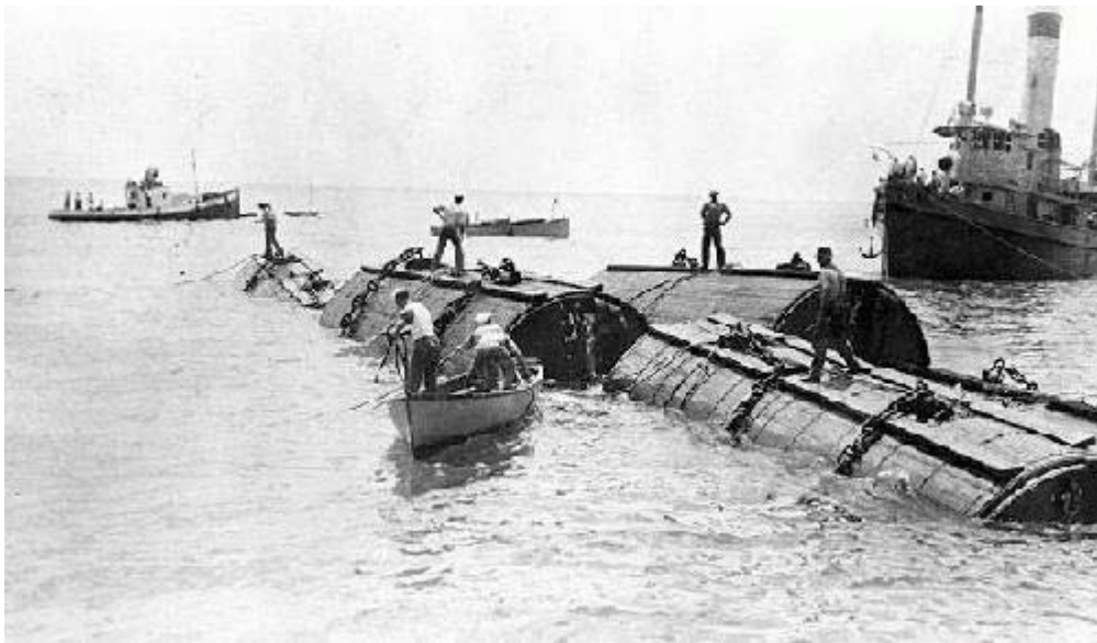
(4) Hole in hull is examined. The port bow plane can be seen in the foreground.
